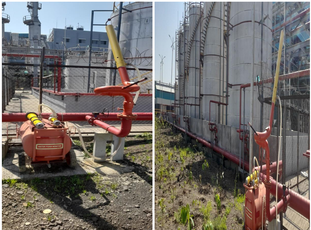
Water cum foam monitors provided at PESO & MEG tankfarm
